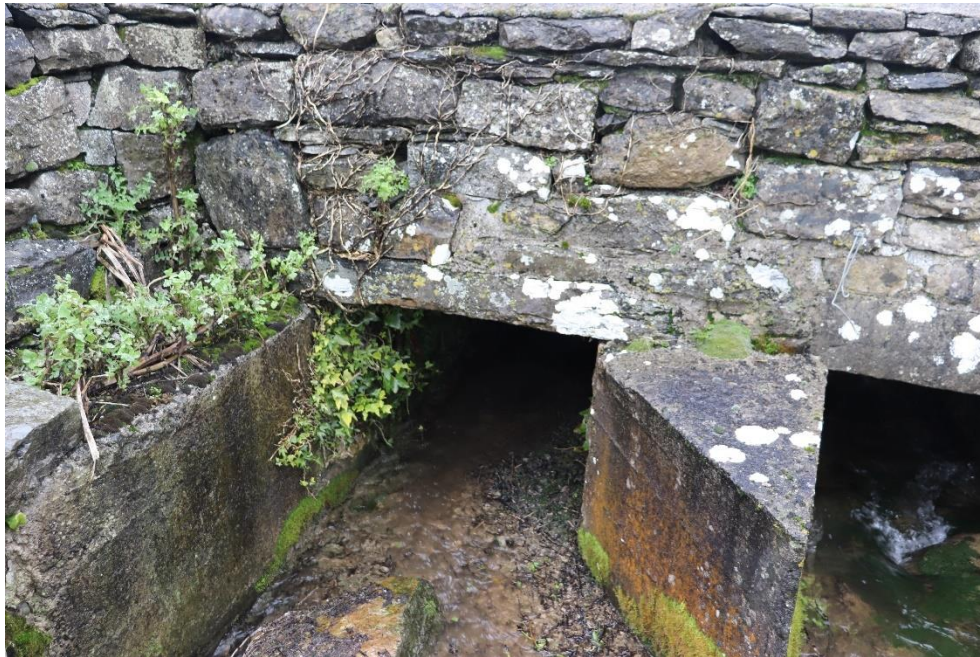
Figure 44 – Transverse Capping Stone on Northern Culvert
