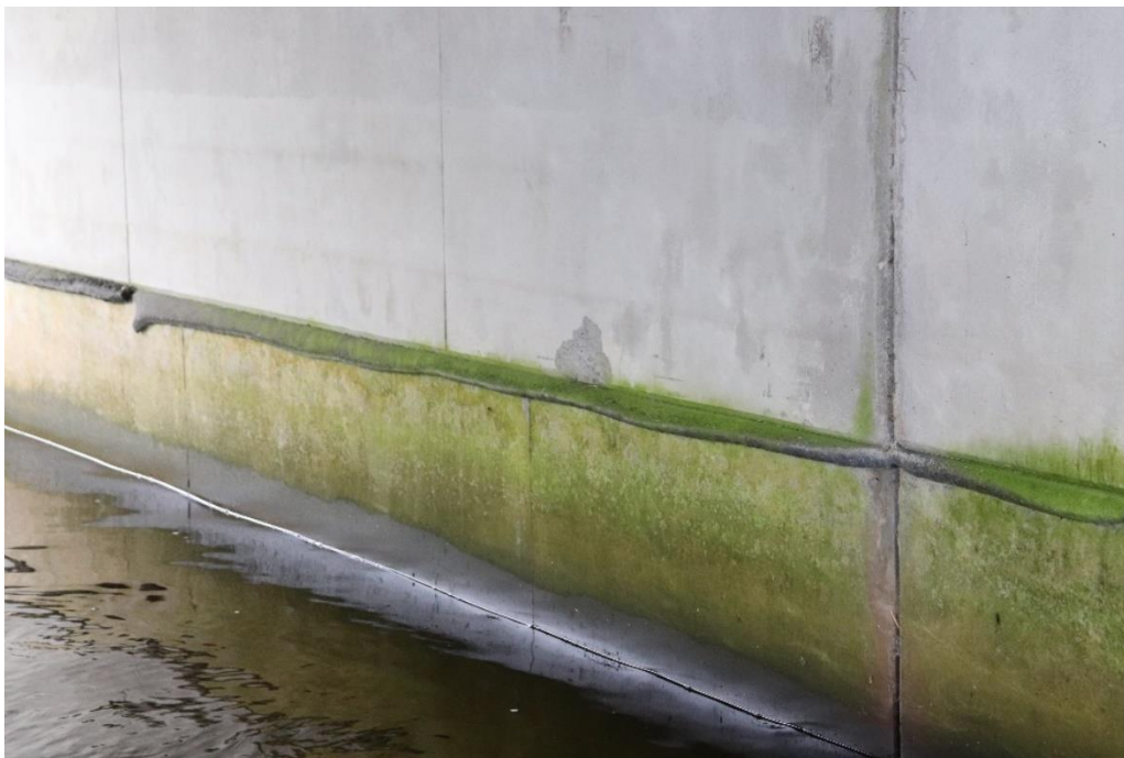
Figure 25 - Spalling of Concrete on North Abutment
