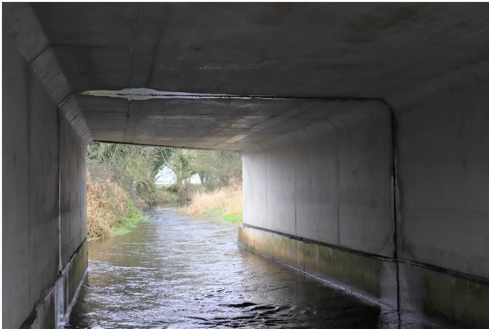
Figure 13 - Central Span Internal
