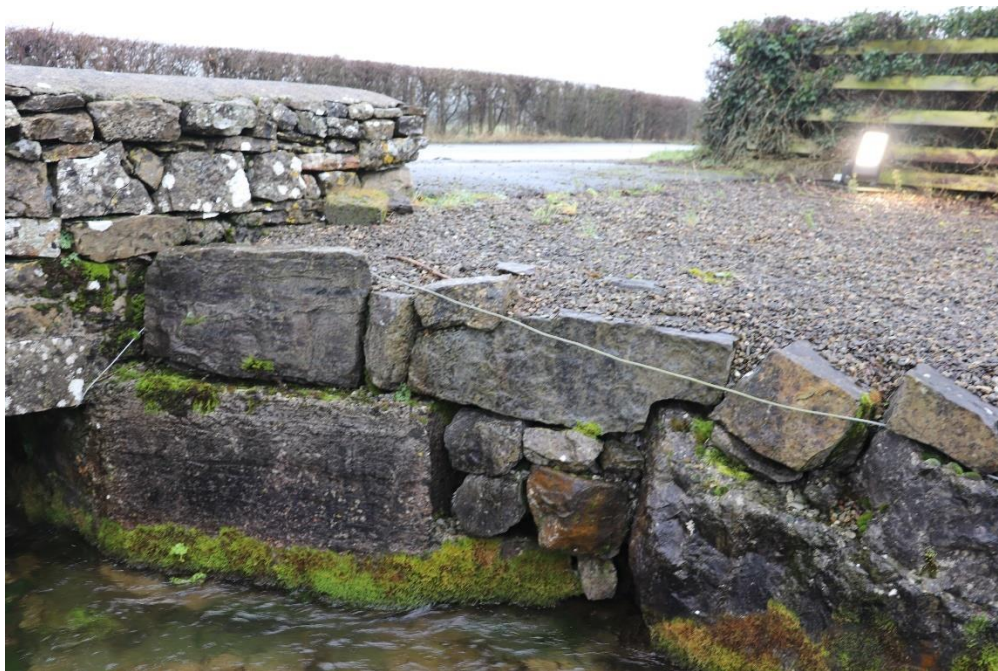
Figure 40 – Southwest Wingwall and Abutment
