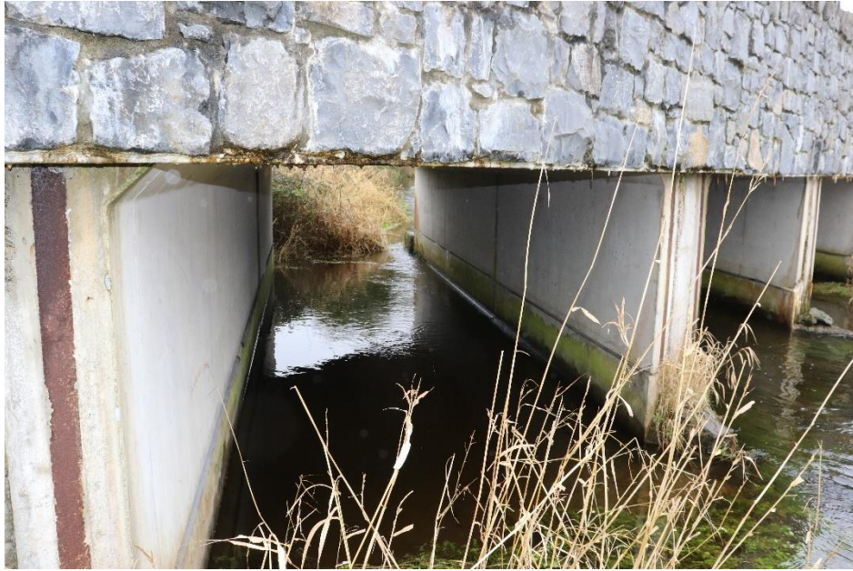
Figure 9 - South Span External
