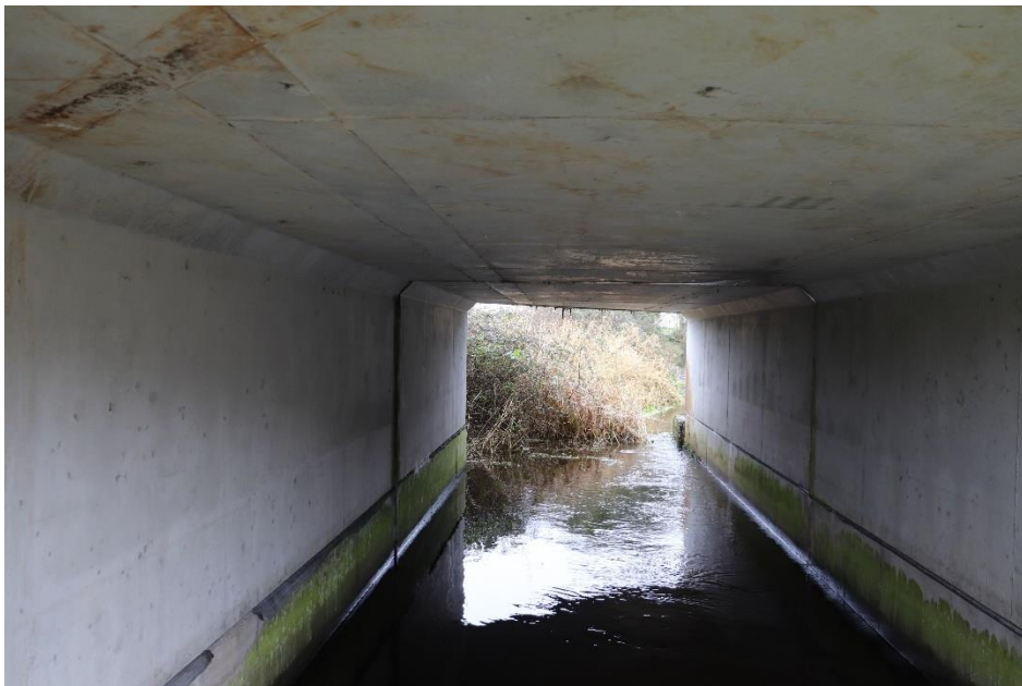
Figure 10 - South Span Internal
