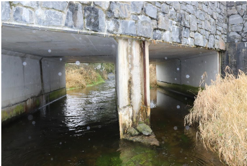
Figure 12 - North Span, Central Span and South Pier
