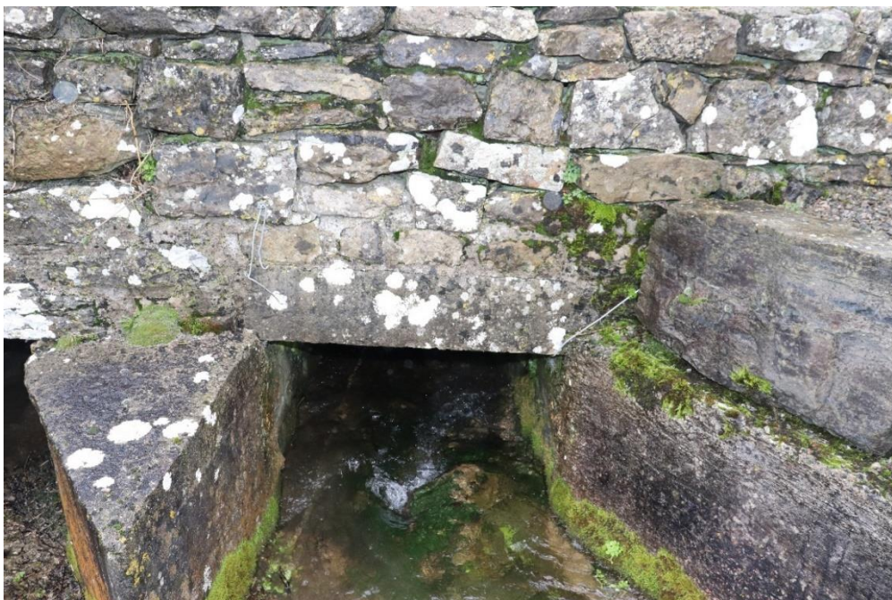
Figure 42 – Transverse Capping Stone on Southern Culvert
