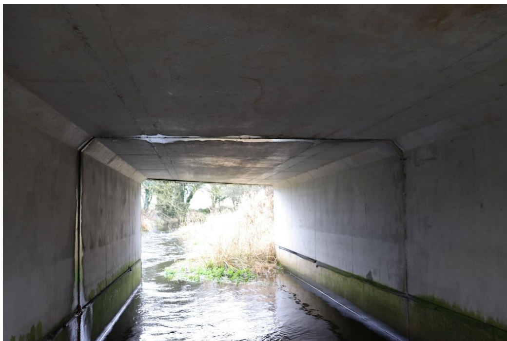
Figure 14 - North Span Internal
